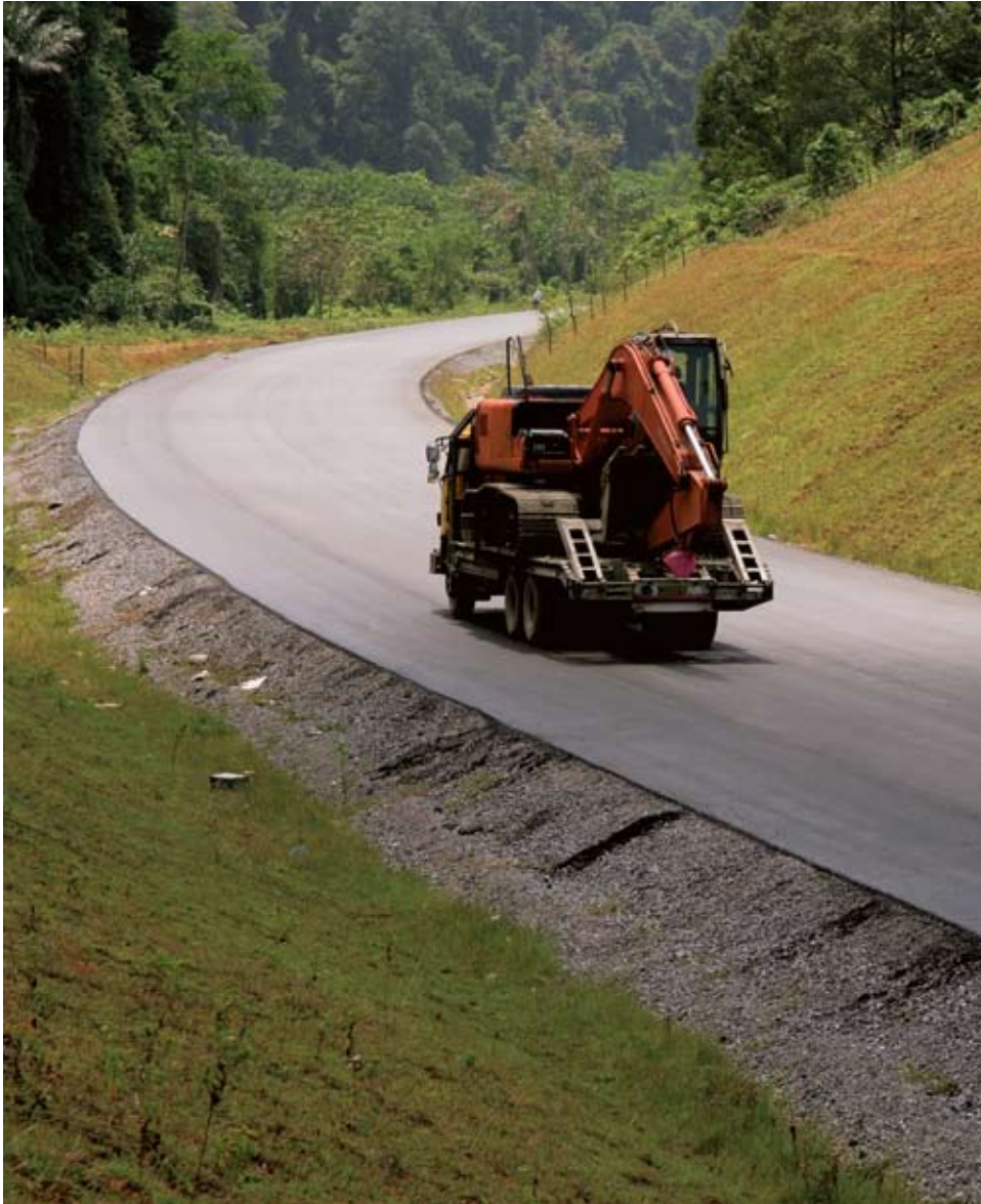
A truck carrying an excavator travels along a well-constructed road in Lhoong, Aceh Besar. The Lhoong road is a section of the Banda Aceh-Calang highway which costs around US$240 million and is funded by USAID, having its first stone laid on August 25, 2005. It is hoped that this road will become a trigger for development of the west coast of Aceh which, in turn, will bring it to catch up with the development of the east coast. Photo: BRR/Arif Ariadi
