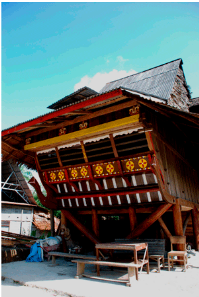
Traditional Nias house after rehabilitation. Photo: ADB Documentation
